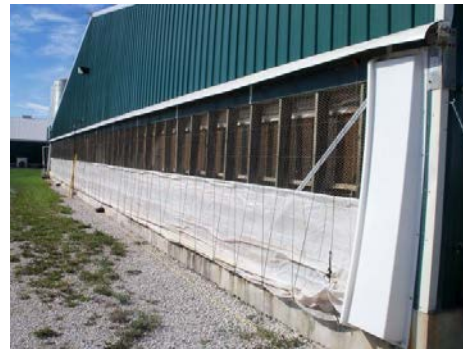
Figure 1. Evaporative cooling pad in the monitored swine gestation barn with curtain half open.
