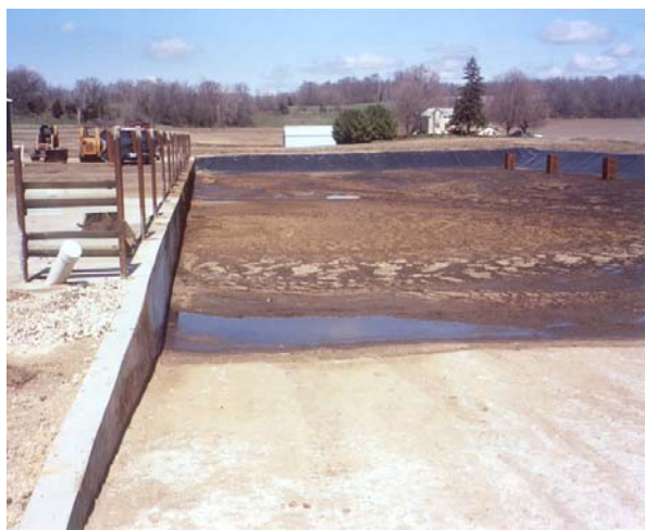
Figure 1. Scraper loading of sand-bedded dairy manure storage.
