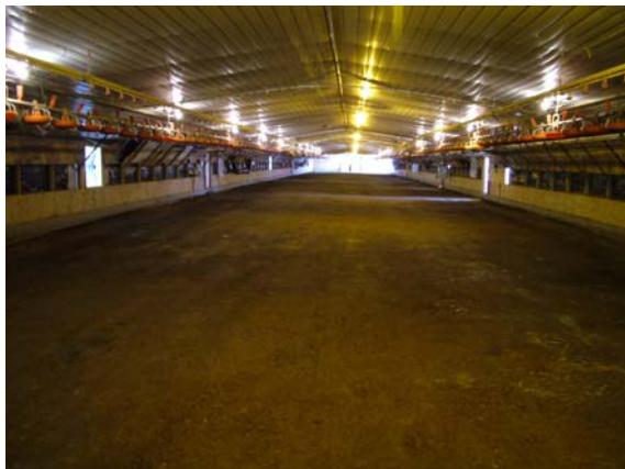
Figure 3. Inside view of one of the broiler houses.
