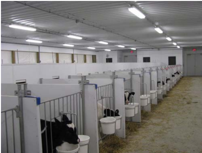
Calf barn: 96 head; rock drainage with geotextile fabric
