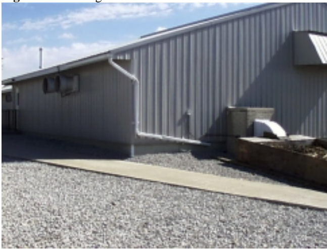
Figure 1. Building site well maintained.
