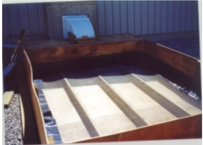
Picture 3: Plastic inside filter forces air away from sides.
