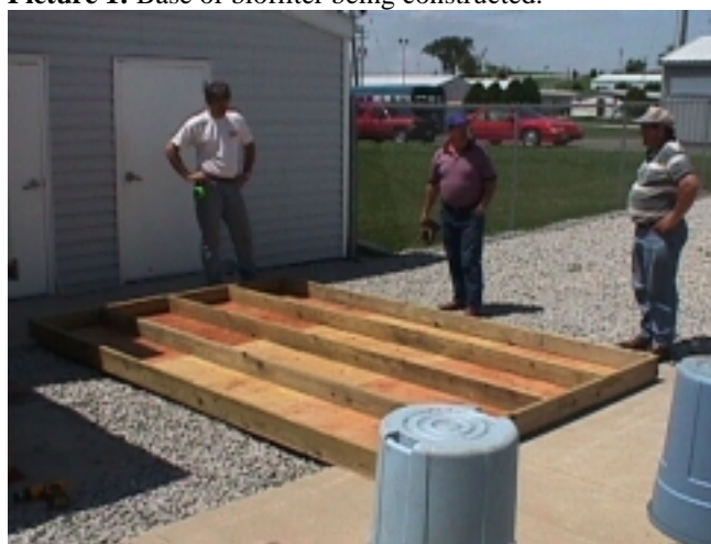
Picture 1: Base of biofilter being constructed.
