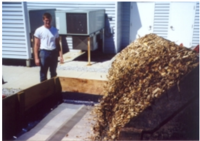
Picture 4: 75% compost and 25% wood chips added to the biofilter.
