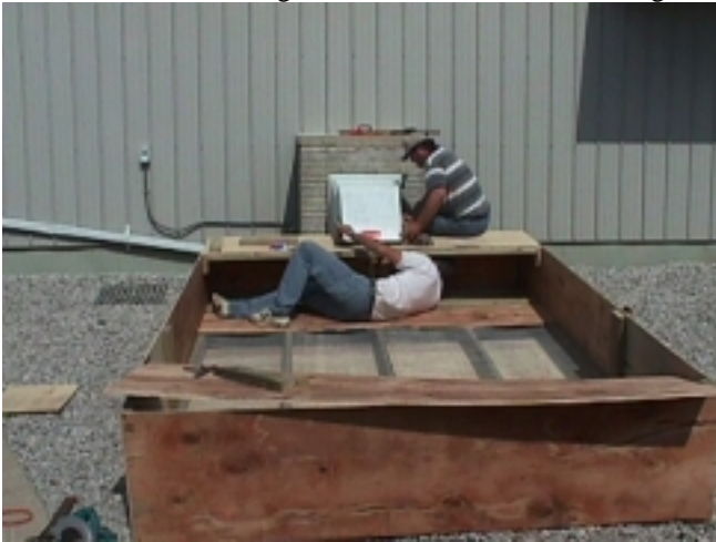
Picture 2: Plenum being attached to exhaust fan housing.
