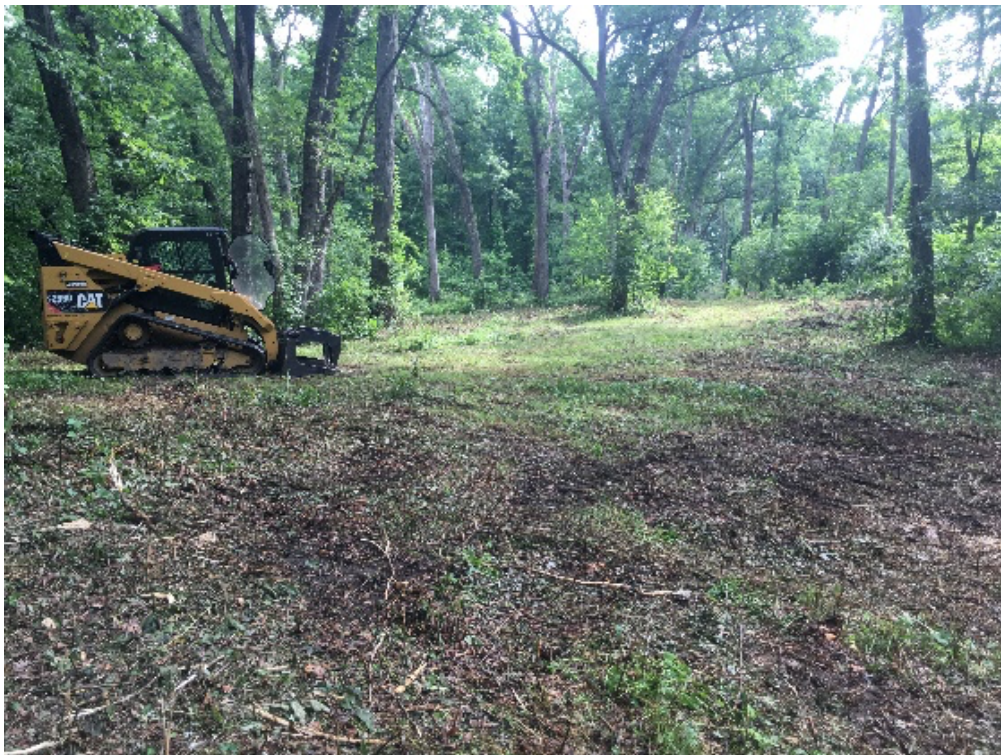
Figure 2. Site preparation for future oak and black walnut direct seeding. Site prep activities included mowing and herbicide spray treatment of multiflora rose and prickly ash, and removal of large debris to allow for equipment access.
