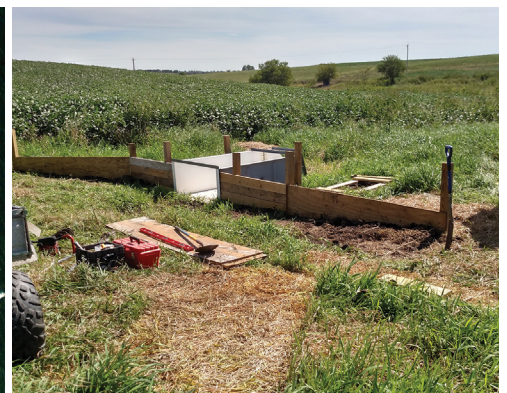
Figure 2: Flume structure for monitoring runoff.
