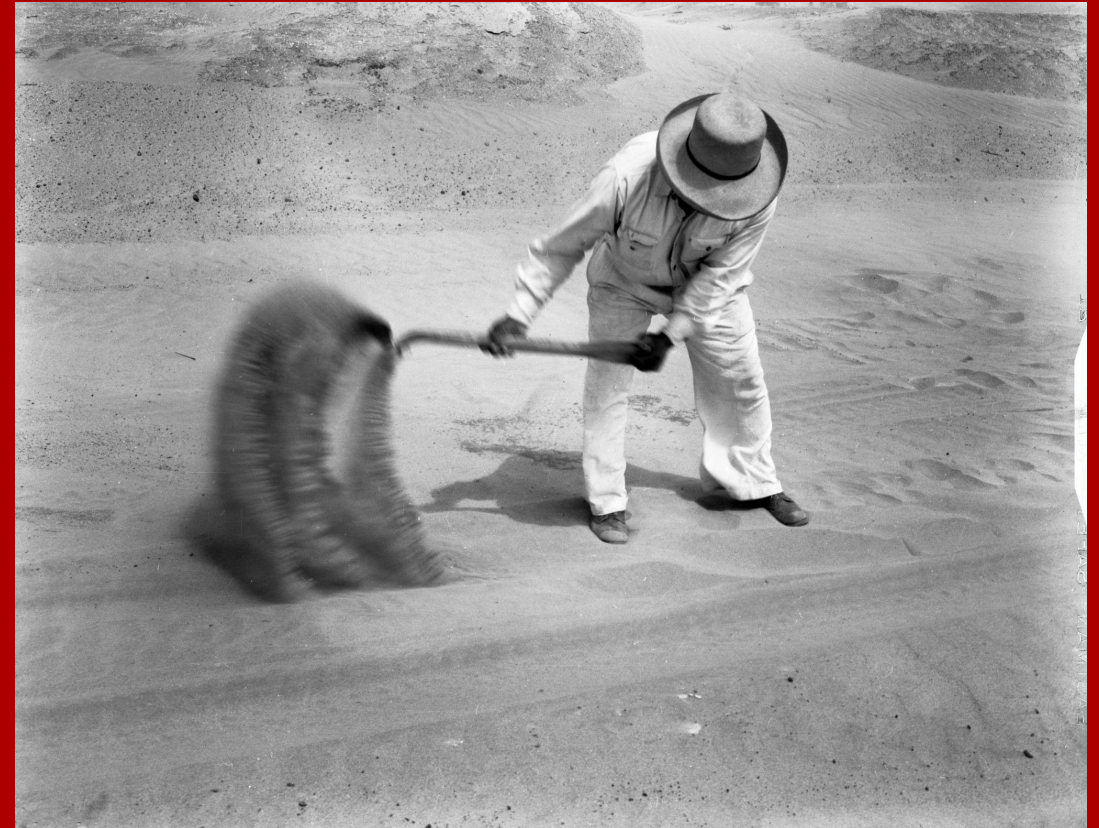
Collier, John Jr. Worker clear buried railroad track, Talara, Peru, 1945 . Oct. 1945. Talara (Piura, Peru). University of Louisville Archives & Special Collections ULPA SONJ_32765
