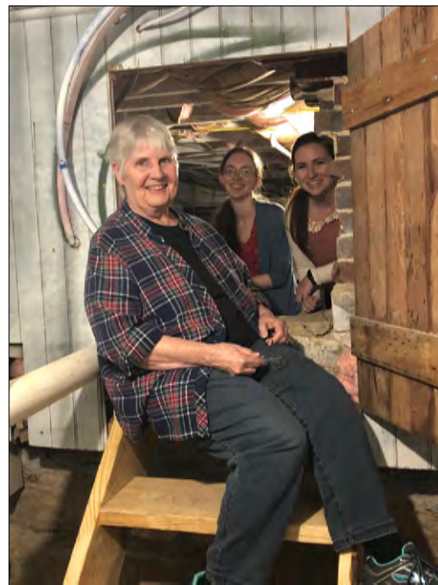
Heritage Center Staff explore the crawlspace. From left to right: Executive Director Eleanor Craig, SL; Curator Susanna Pyatt; Archivist Ayla Toussaint.
