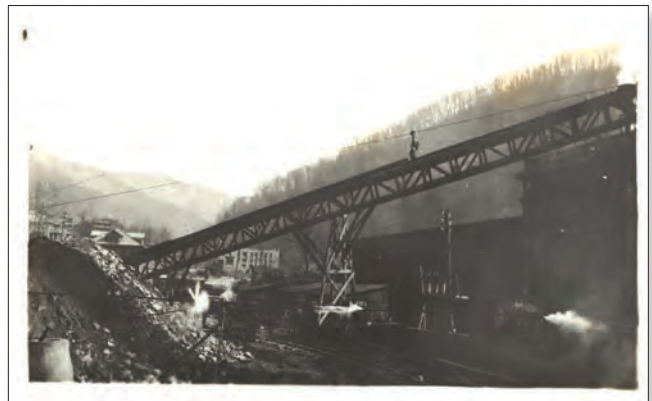
A worker standing on a coal mining belt, surrounded by the Appalachian Mountains, page 27. Courtesy of The Filson Historical Society.
