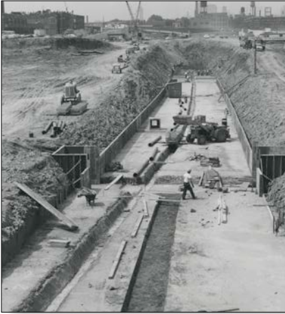
Construction of expressway in Chicago, circa 1961
