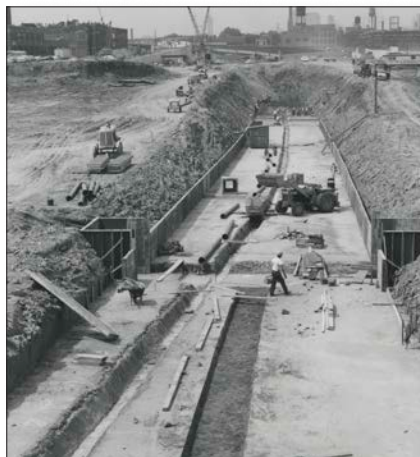
Construction of expressway in Chicago, circa 1961
