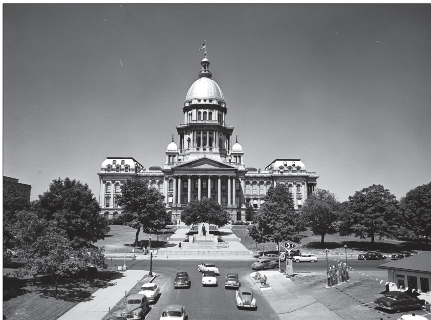
Doc Helm photographed the Illinois Capitol Building in 1947.
