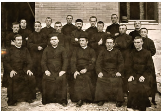
The first SVDs during construction of their community in Techny, IL, 1900
