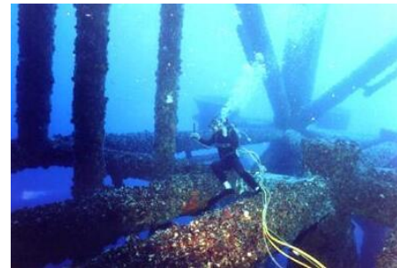
Fig. 1. Attachments on underwater structure
