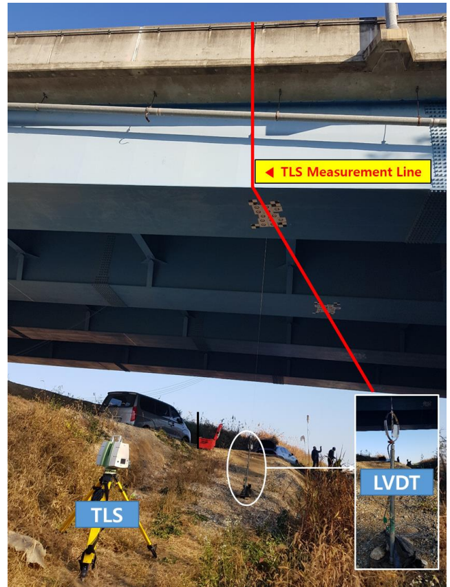
FIGURE 2: LASER SCANNING MEASUREMENT EXPERIMENTS FOR NOSEONG BRIDGE
