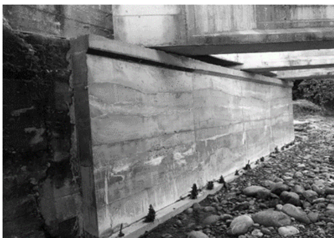
Figure 2. Palomas Bridge reinforcement.
