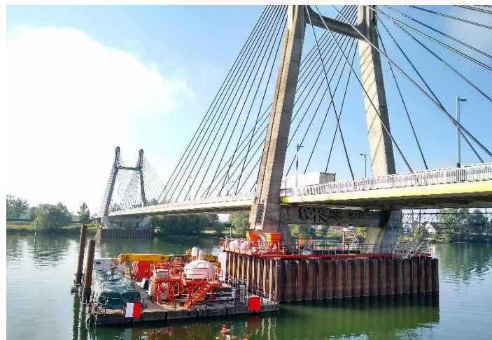
Figure 1: General view: pylon base repairing works
