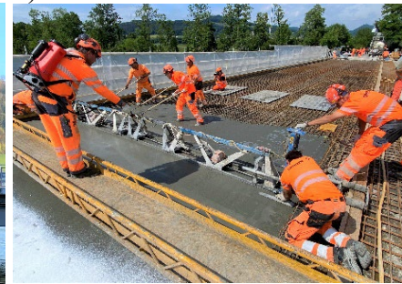
Figure 6 a) View of the steel-concrete composite bridge after R-UHPFRC strengthening, b) casting of UHPFRC with immediate application of curing compound.
