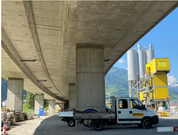
Figure 5 a) UHPFRC ready mix plant next to the Riddes Viaduct, b) UHPFRC casting on the deck slab.
