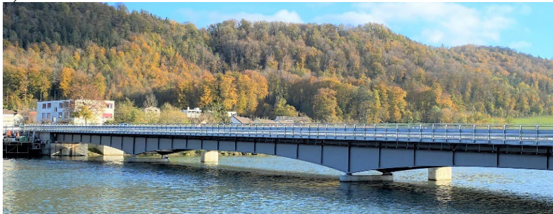
Figure 6 a) View of the steel-concrete composite bridge after R-UHPFRC strengthening, b) casting of UHPFRC with immediate application of curing compound.
