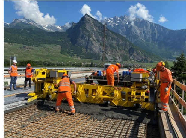
Figure 5 a) UHPFRC ready mix plant next to the Riddes Viaduct, b) UHPFRC casting on the deck slab.
