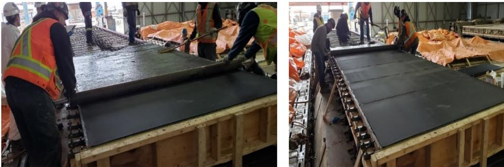
Figure 4: Smoothing the Concrete Surface (left) and Placing Ribbed Matting (right)
