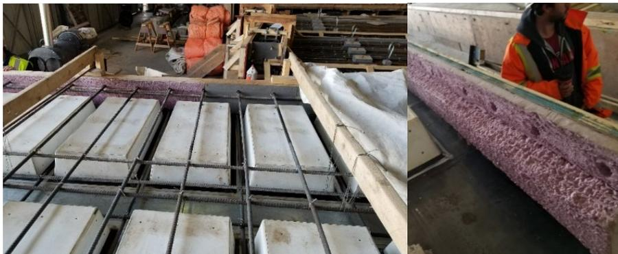
**Figure 2: Photographs of Full-Scale DIB Formwork**
