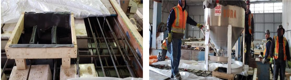
Figure 3: Chute for Casting (left) and Transport Bucket Loading Chute (right)
