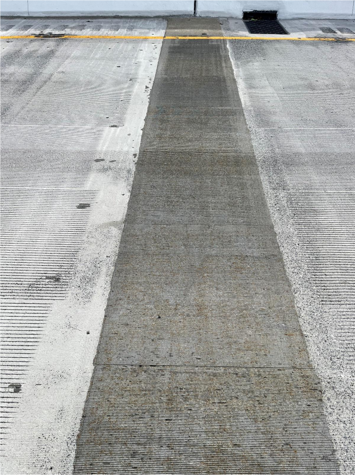
Photo 2: Completed Link Slab
