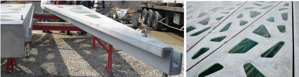
Figure 2: Principle of fitting triangular tiles with side channels for the roofing of Jean Bouin Stadium
