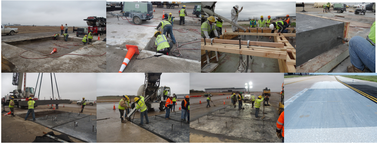
Figure 2: Implementing UHP-FRC precast panels, surface roughening, and onsite UHP-FRC joint grouting
