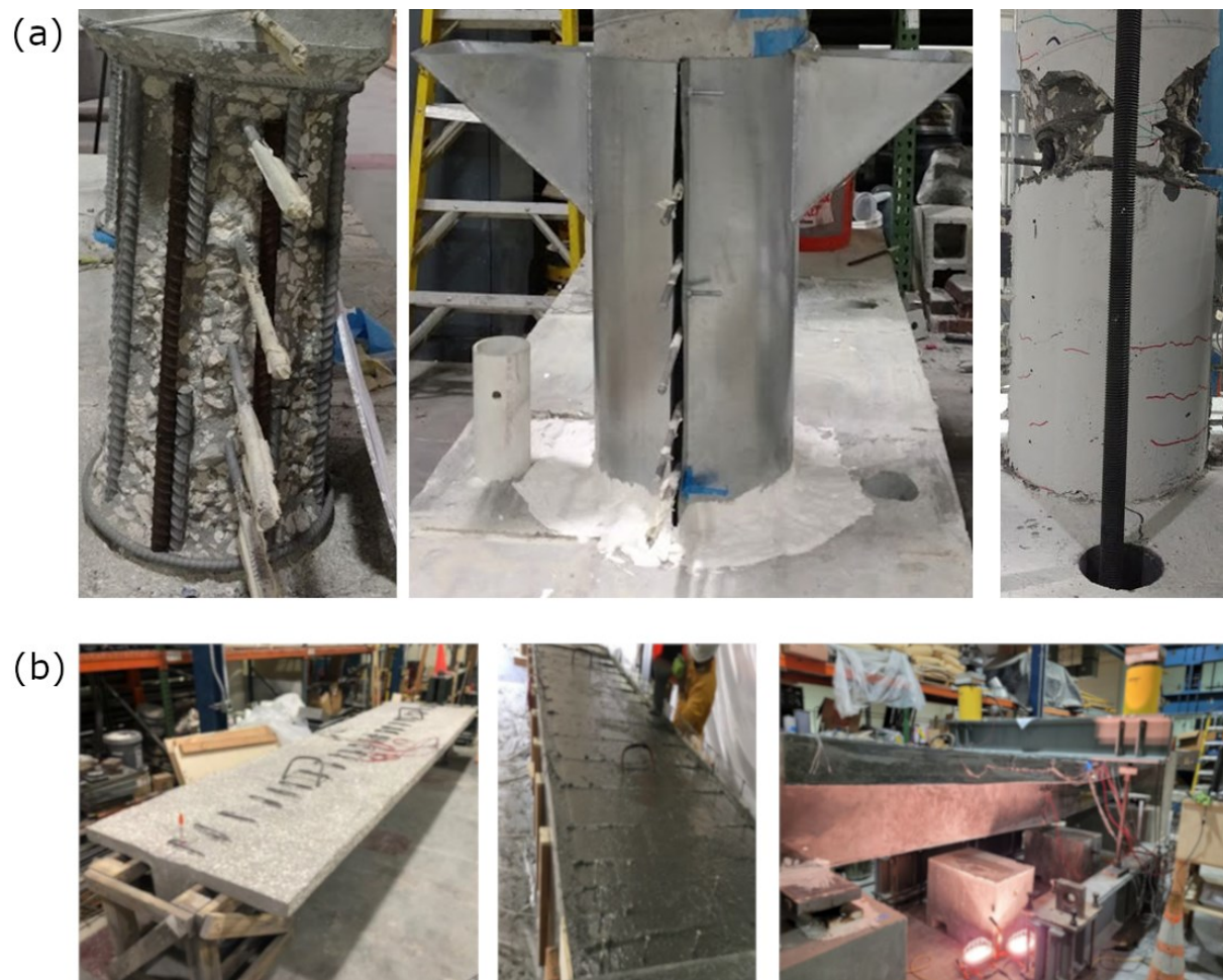
Figure 2. Using UHPC to retrofit bridge elements: (a) retrofitting column specimen (Farzad, Shafieifar and Azizinamini), (b) retrofitting beam specimen (Valikhani and Azizinamini).
