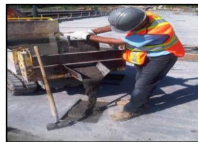
Figure 5: Filling the joints with UHPC
