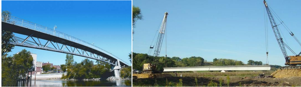
Figure 2: a) (Left) Sherbrooke Pedestrian Bridge, Quebec, Canada (1997); b) (Right) Placing UHPC I-girders at Mars Hill Bridge, Wapello County, Iowa, USA (2006).
