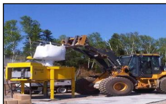
Figure 4: UHPC Portable Mixers
