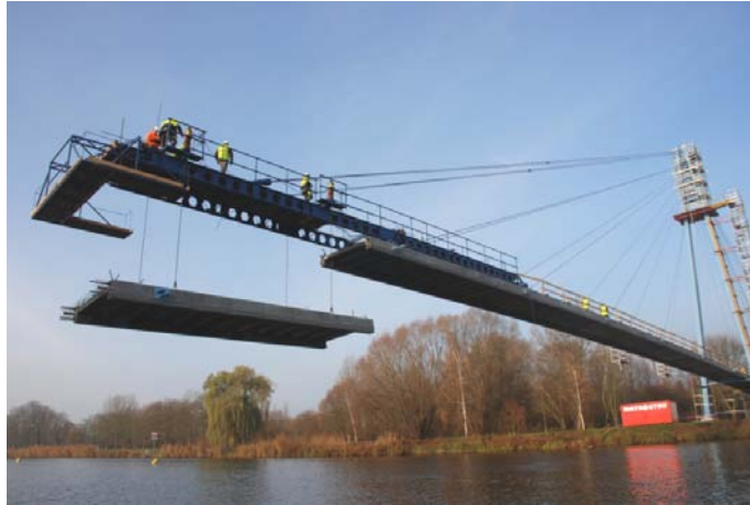
Figure 6: Assembly of the segments over the river using a launching gantry
