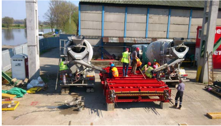
Figure 4 – Segment mould filling by UHPC flowing from truck mixers
