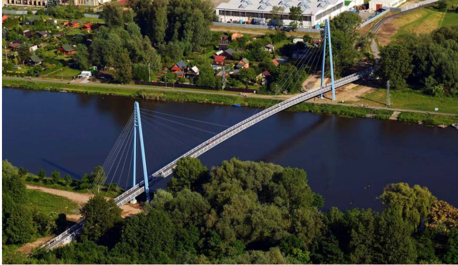
Figure 7: The completed footbridge
