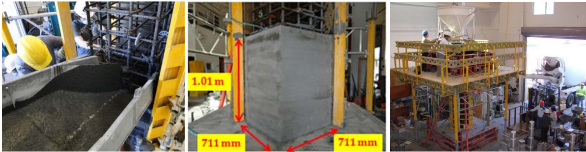
Figure 4. UHP-FRC (a) Pouring and (b) Completed Section (c) Final Casting
