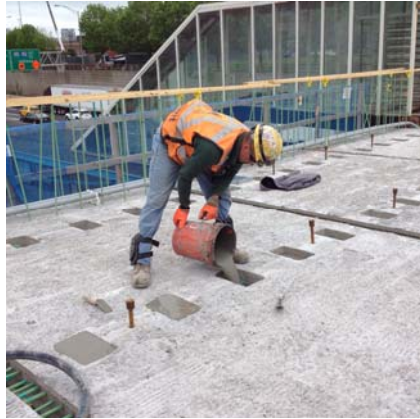
Figure 7. Casting of Non-Shrink Grout at Shear Stud Pockets
