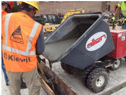
Figure 8. Casting of UHPC
