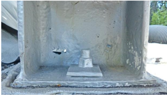
Figure 13. Corrosion at the base of a bent leg. Figure 14. Bents with formwork for encasement.
