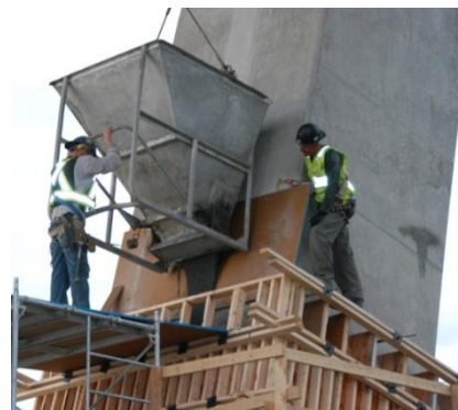
Figure 8. Placing via top of the form
