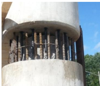
Figure 10. Existing rebar and new dowels
