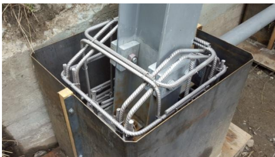
Figure 15. Reinforcing rebar cage and steel bolted to the flange leg
