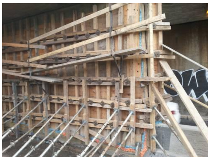
Figure 3. Formwork ready for casting
