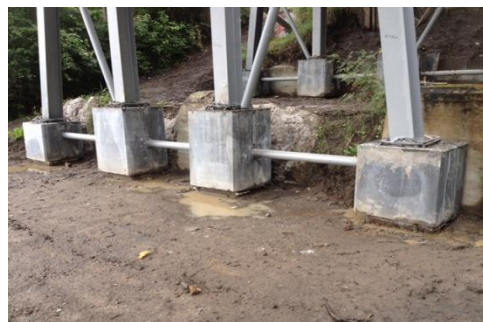
Figure 16. Ductal ® encasement of the bent plates bases prior to capping
