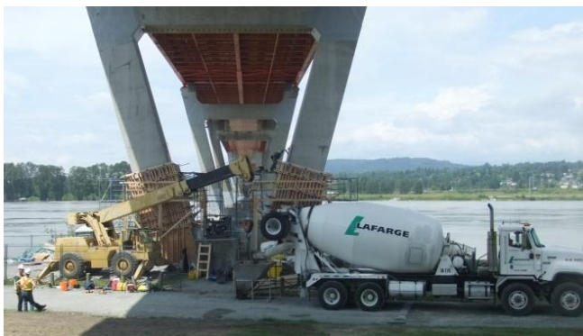
Figure 7. Batching / delivery to site by ready-mix trucks
