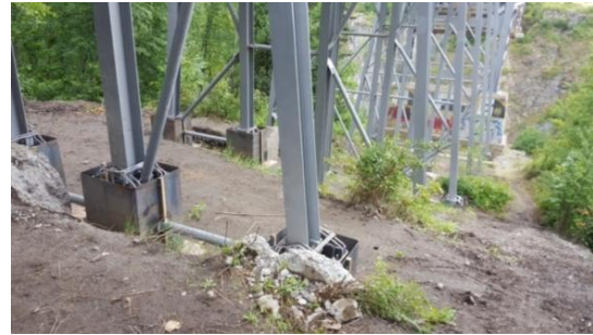
Figure 13. Corrosion at the base of a bent leg. Figure 14. Bents with formwork for encasement.
