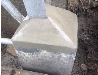
Figure 17. Ductal ® encasement capped for drainage with zero slump mortar
