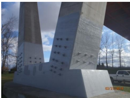
Figure 5. Existing prior to final retrofit
