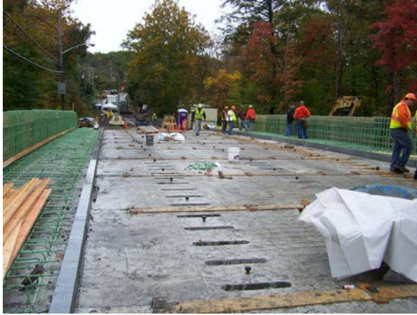
Figure 3–Case Study 3-Route 42 over Westkill Panel Joint Placement in Progress
