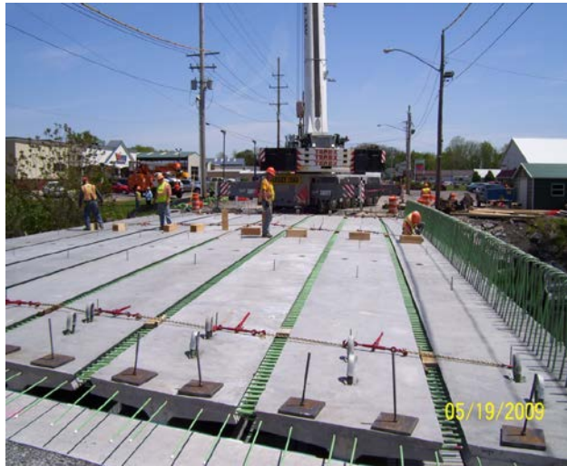
Figure 1–Case Study 1–Rte. 31 over Canandaigua outlet DBT in place before UHPC placement
