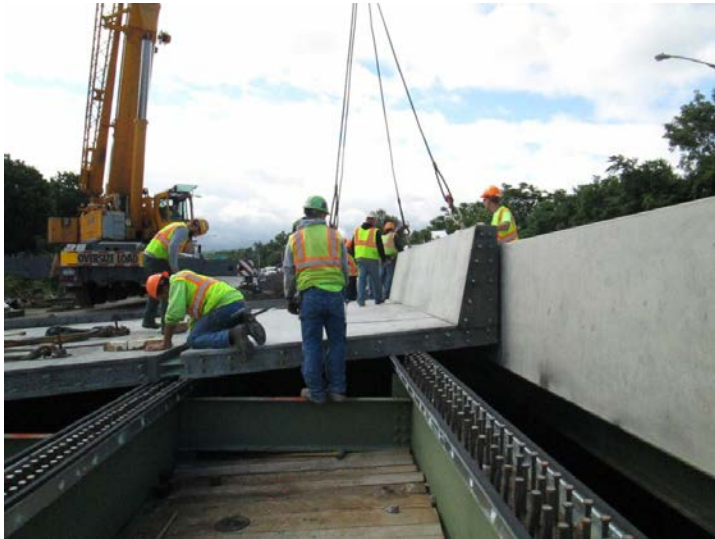
Figure 4-Case Study 4 – I-81 over East Castle St. Precast Deck Placement in Progress
