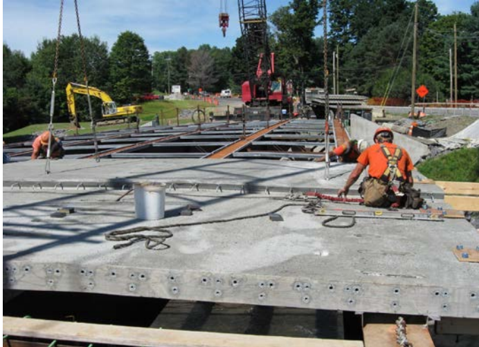
Figure 2–Case Study 2-Route 23 over Otego Creek in Oneonta Precast Deck Placement in Progress
