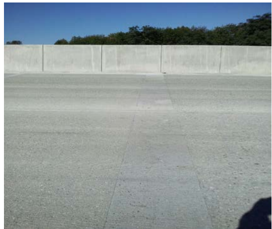
Figure 6-Finished Link Slab
