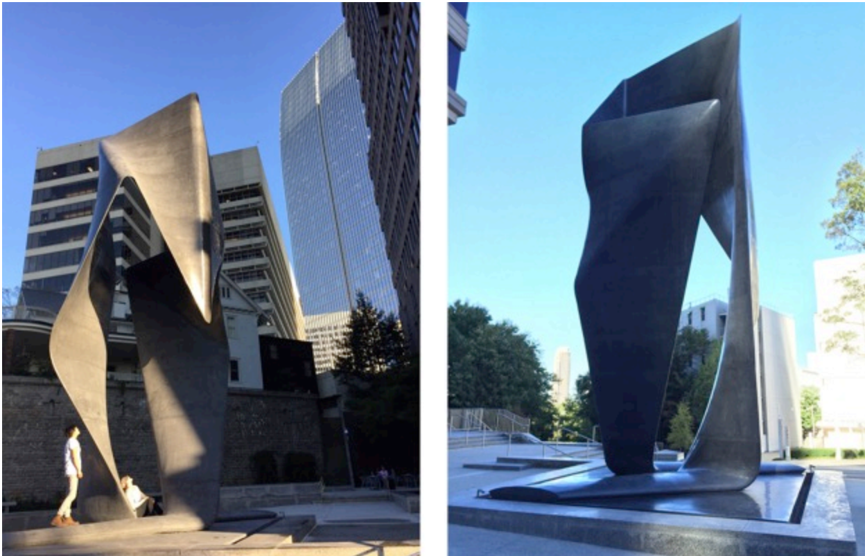
Figure 1: Stealth Sculpture in Reinforced Concrete
