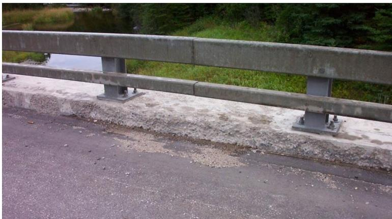
**Figure 1.** An Example of Premature Concrete Deterioration on an MTO NWR Project
