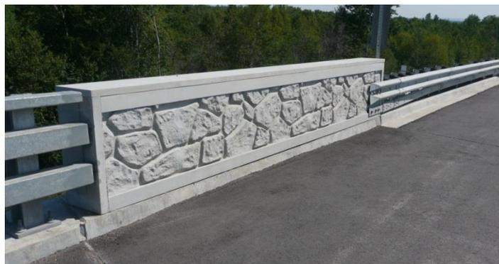
**Figure 8.** UHPC Barrier Endwall Treatment
