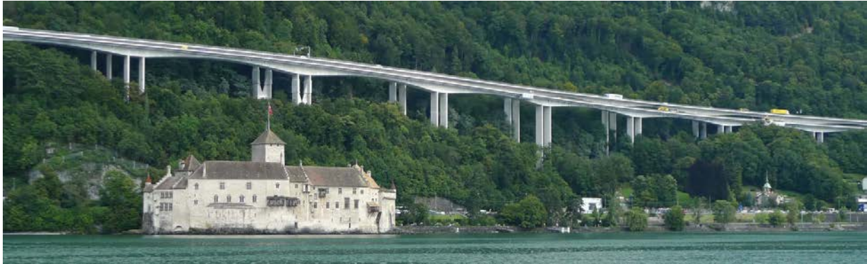
Figure 5. Chillon Viaducts along Lake Geneva.
