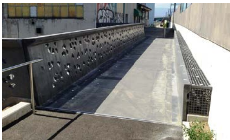
Figure 8. Martinet Pedestrian Bridge in Lausanne, Switzerland; Top: overall view of illuminated bridge at dusk, Middle: “organic” web and bottom plate with ribs, Bottom: asymmetric cross section (dimensions in mm).
