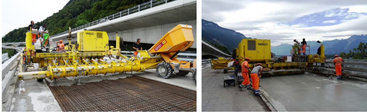
Figure 7. UHPFRC casting machine (left), and fresh UHPFRC layer after casting (right).
