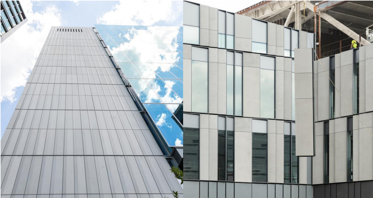
Figure 1 – Examples of UHPC Facades in the USA: (a) 860 Washington, New York City (b) University of Cincinnati, Lindner College of Business.
