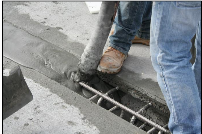
Figure 4. UHPC Being Successfully Placed with a Pump in Late Autumn of 2014
