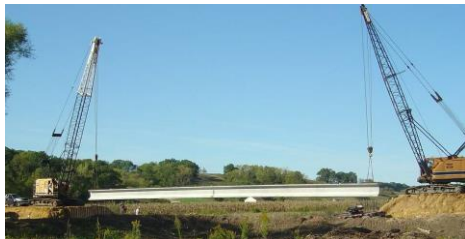
Figure 3: Placing a UHPC I-Girder
