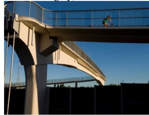
Figure 2: Glenmore/Legsby Pedestrian Bridge
