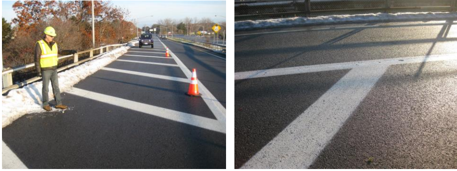
Figure 12. No reflective cracking on top of UHPC link slab
