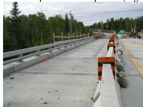
Figure 6. Rainy Lake Bridge Deck - Phase 2
