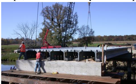
Figure 4: Installation of 2 nd Generation Pi-girder
