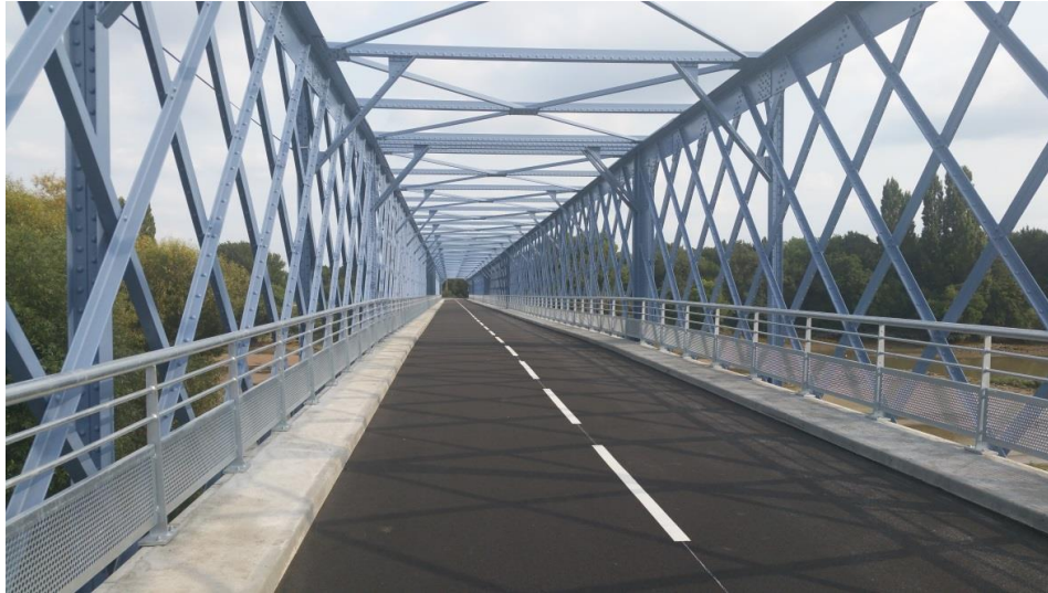
Figure 13: Picture of the finished bridge
