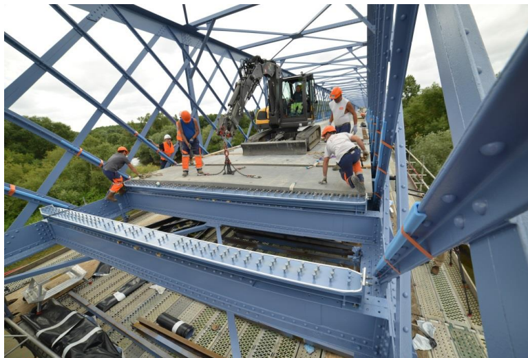
Figure 10: Picture of a slab installation.
