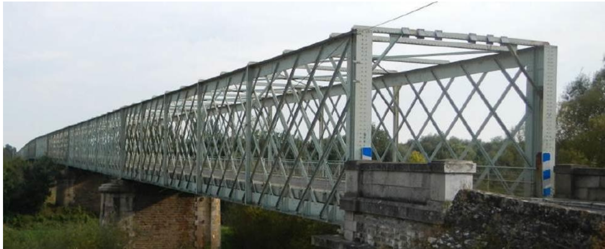
Figure 1: General view of the bridge before renovation
