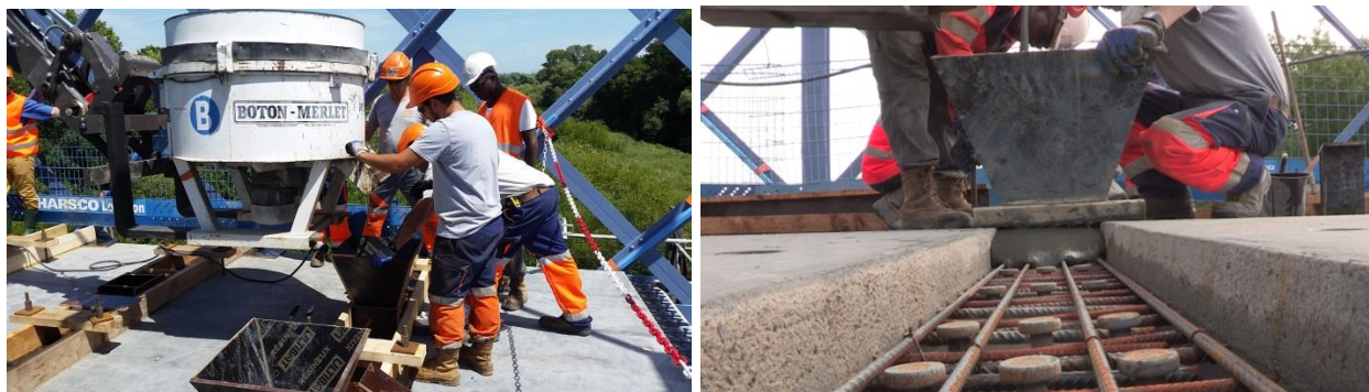
Figure 12: Pictures of a UHPC connection realization
