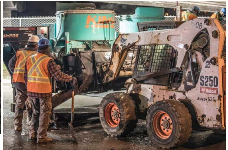
Figure 2 - UHPFRC discharged in mixer
