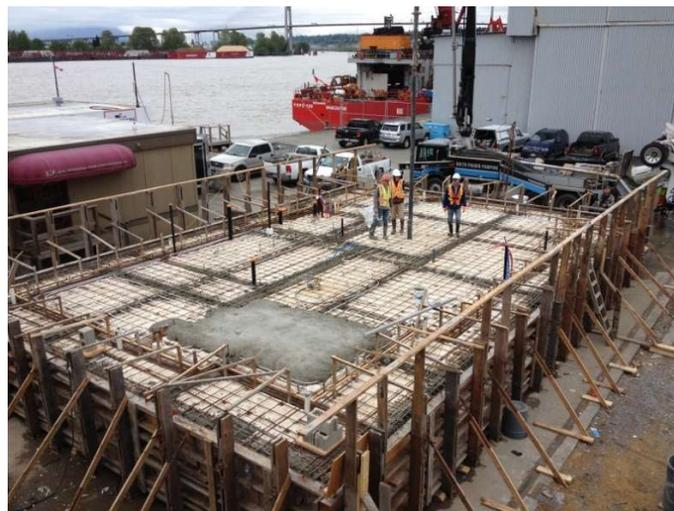
Figure 2 – Concrete Floating Foundation with EPS Foam (Peters, 2013)
