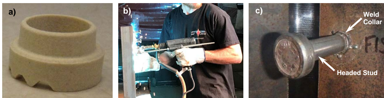
Figure 3. Welding of headed shear studs including a) ferrule, b) welding on a vertical plate, and c) finished product.
